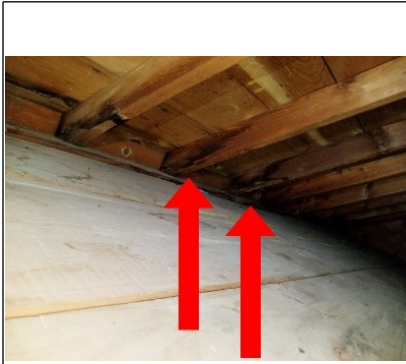
Moisture stains. There are no ventilarion on this side of attic.
